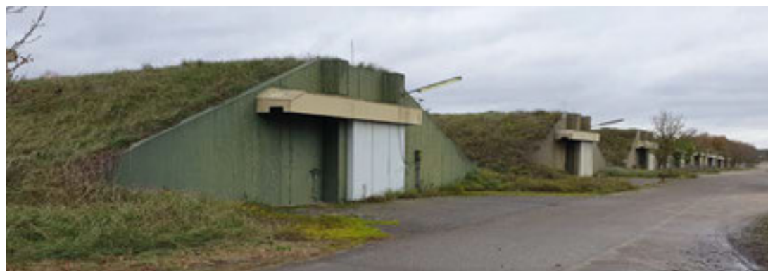
Figure 10.3 NATO bunkers (Source: Amsterdam Office for Serious Fraud, Environmental Crime and Asset Confiscation)
